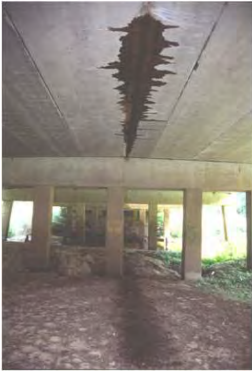
Photo 7: Staining along longitudinal joint. Note guano deposits on the ground. Photo 8: Staining on underside of expansion joint from bat use.
