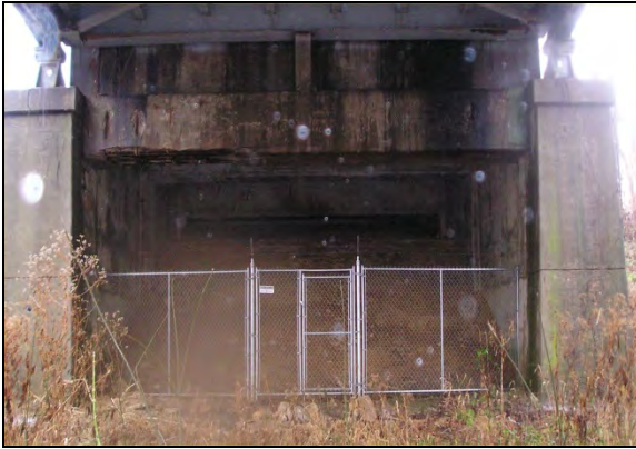
Photo 12 and 13: Bridge Design Mimicking “Cave-like” Atmosphere
