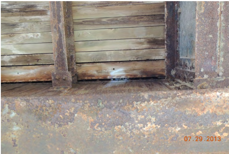
Photo 14: NLEBs Roosting Under a Timber Decked Bridge
